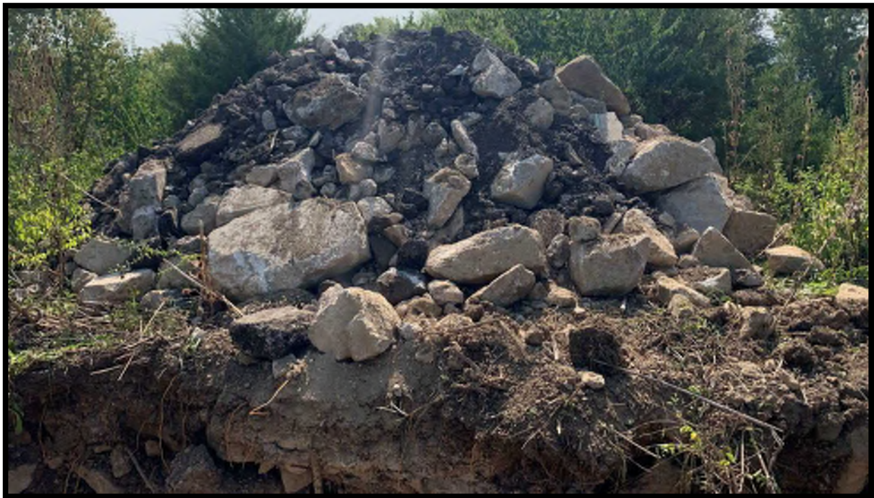
Test Pit TP-2 Spoils
