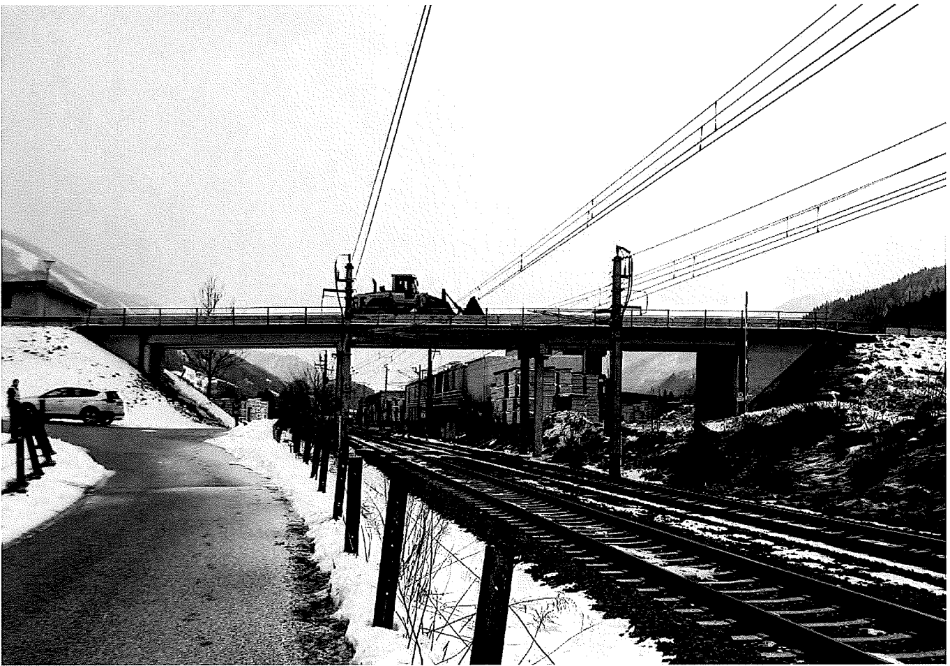
A view of the railway bridge in Austria previously damaged by heavy timber transportation – now protected thanks to the KiTraffic Statistics Weigh In Motion (WIM) system from Kistler
