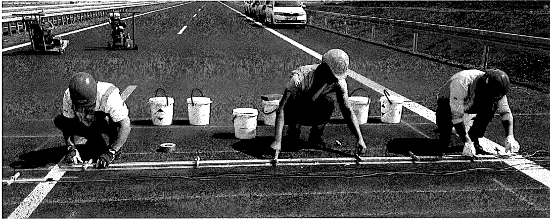
Installation of Lineas sensors in the road
