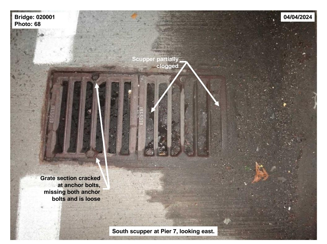
Replaced grate loose with cracked tack welds (put back in place during inspection) Scupper partially clogged
