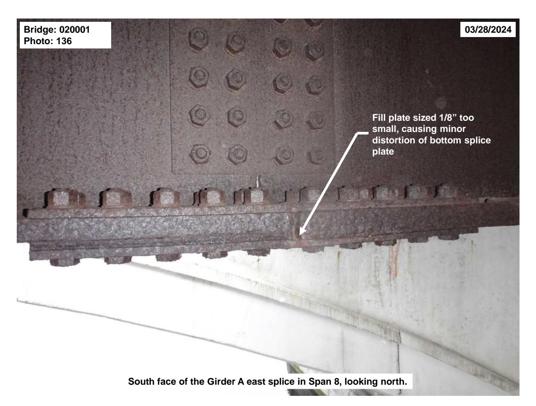
Fill plate sized 1/8" too small, causing minor distortion of the bottom splice plate
