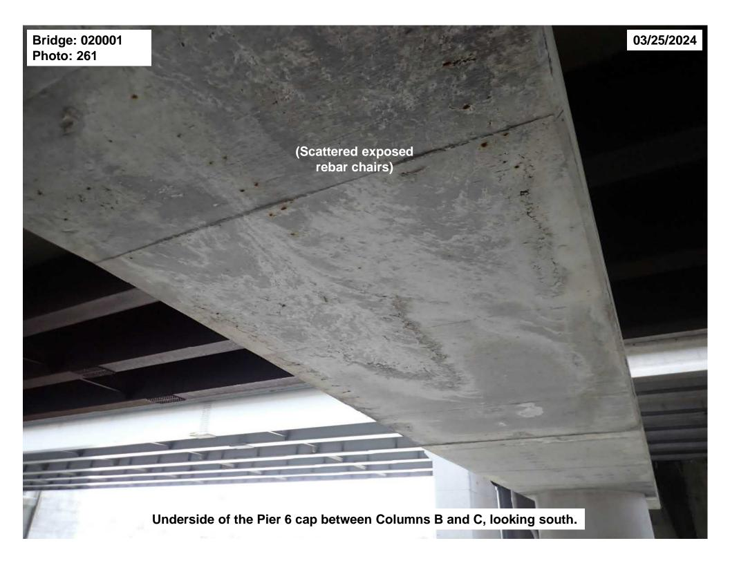
Hairline vertical and diagonal cracks, some with light efflorescence
