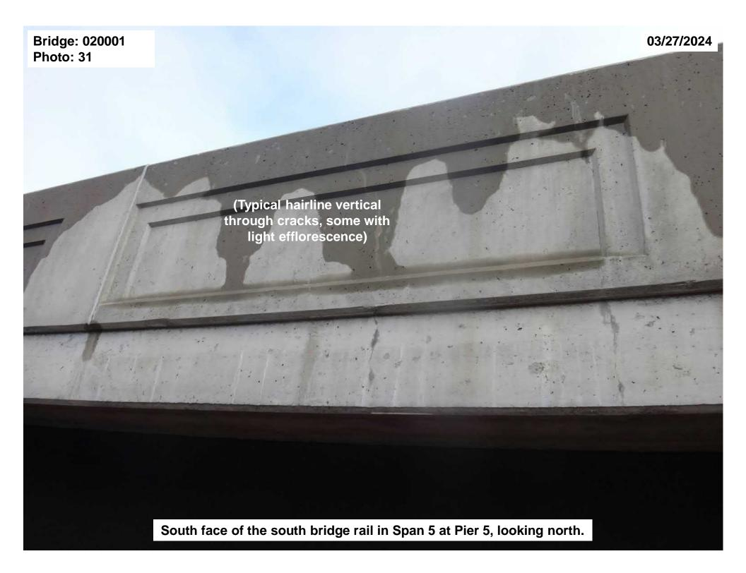
(Scattered full height hairline vertical through cracks, spaced up to 3'-0" apart)
