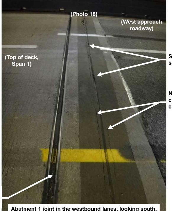
Sections of missing sealant, up to 2'-0" long
