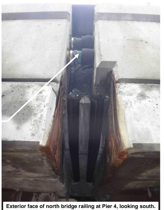
Two (2) conduits at the joint with torn rubber covers
