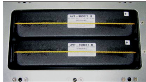
Cover Removed, Exposing 2 Lithium Ion Batteries
