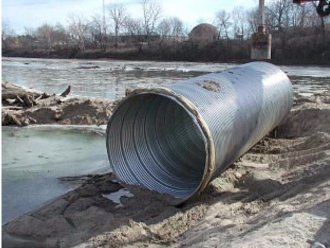
*Note: CMP with burlap to anchor and seal the bottom of the shaft in rock socket and prevent concrete leaking between the casing.*
