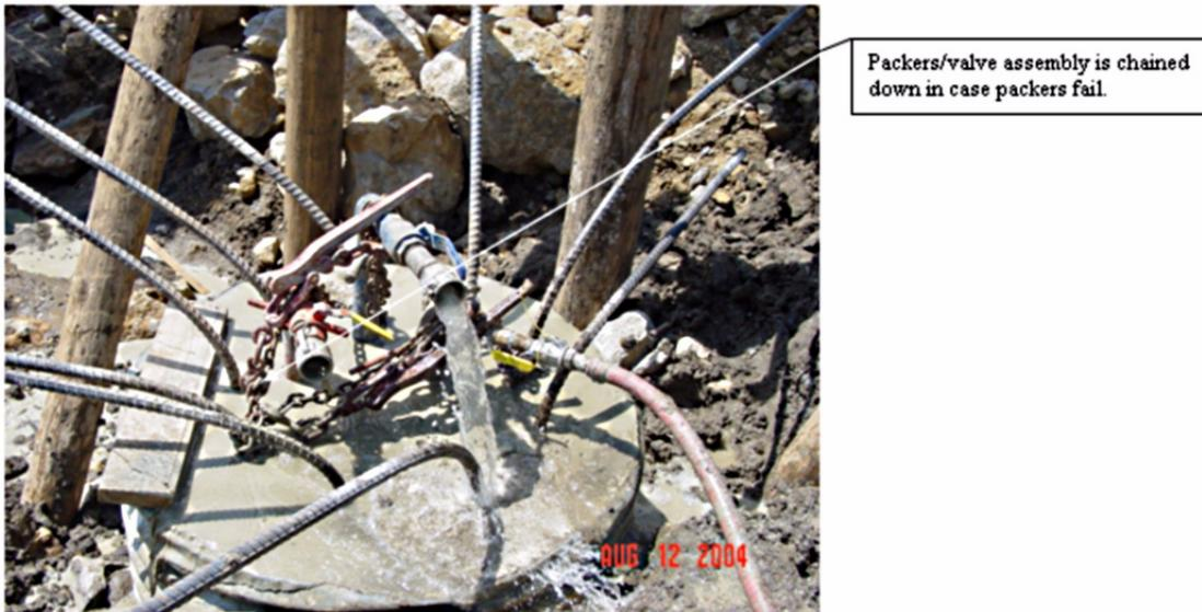
If the void is within the uncased rock socket, care must be taken to prevent “mining” of new material from the side of the hole. This problem exists mostly when the socket is founded in shale or a
