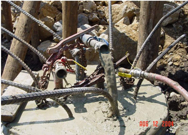
6) Close all exit valves. Pump up the pressure until 20 psi is maintained for 10 minutes. Pressure is applied to ensure that the grout makes it into all of the crevices in the anomaly and coats all of the partially cemented material.
