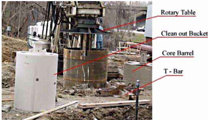
Clean-out Bucket , Rotary Table, T-bar & Core Barrel.
