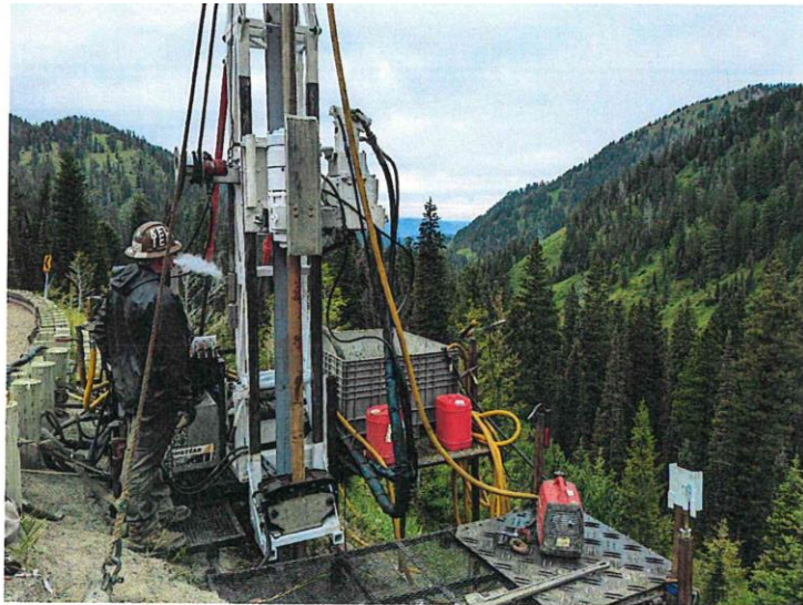
Figure 1: Drill location on embankment slope past the guard rail
